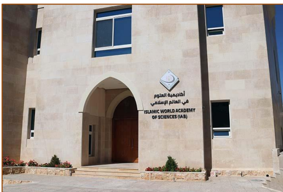
Main Entrance of Building
